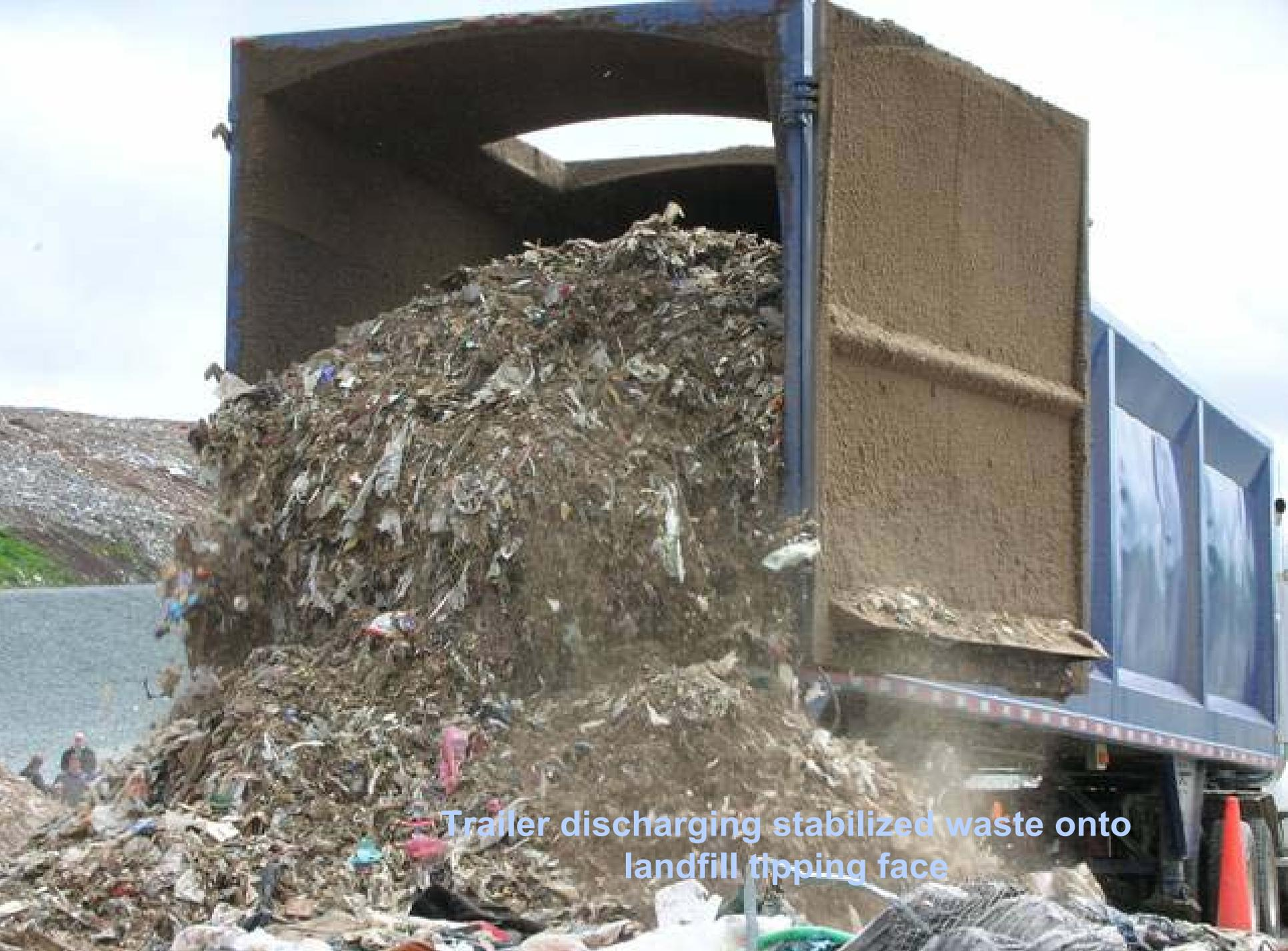
Trailer discharging stabilized waste onto landfill tipping face
