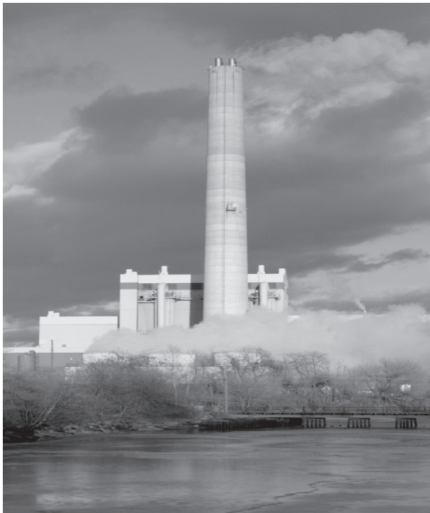
A waste to energy incinerator in Camden New Jersey. Similar projects are being proposed in Ontario
